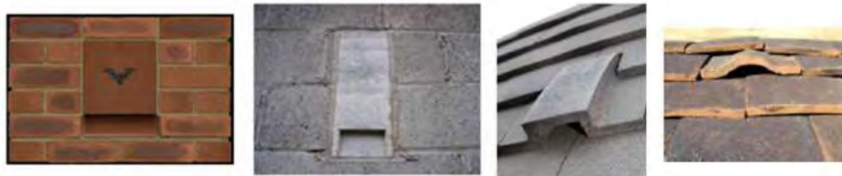
Figure 4: examples of bat tiles, bricks, integrated bat boxes from http://www.bats.org.uk/pages/bat_boxes.html
